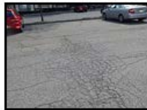
Alligator Cracking
